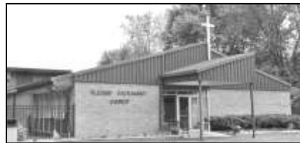
Blessed Sacrament Church and Parish Offices
