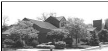
St. John the Evangelist Church, Chapel and Parish Offices
