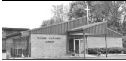
Blessed Sacrament Church and Parish Offices
